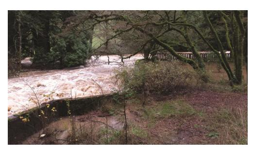
Man-made water structures like this one Johnson Creek can make downstream flooding worse. Metro removed these structures to let Johnson Creek into its wetlands, lowering the risk of flooding in downstream neighborhoods.
